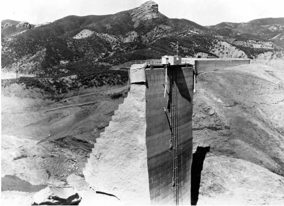
St. Francis Dam, March 17, 1928 (Attribution: U.S. Geological Survey Photographic Library) Figure 4
