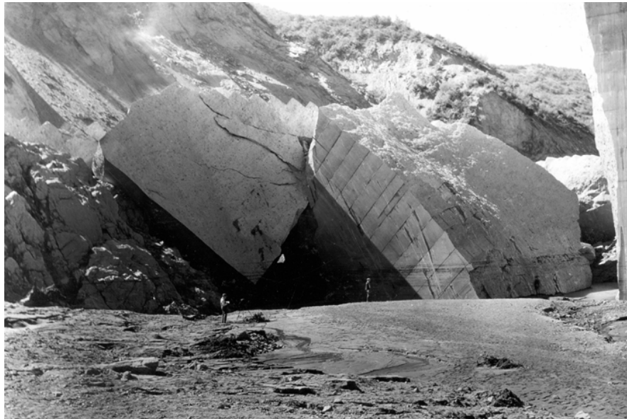
St. Francis Dam, Concrete Debris Blocks (Attribution: U.S. Geological Survey Photographic Library) Figure 5
