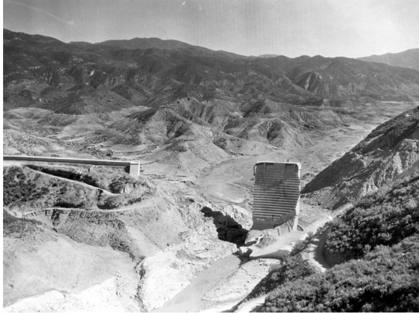
St. Francis Dam, March 17, 1928 (Attribution: U.S. Geological Survey Photographic Library) Figure 3
